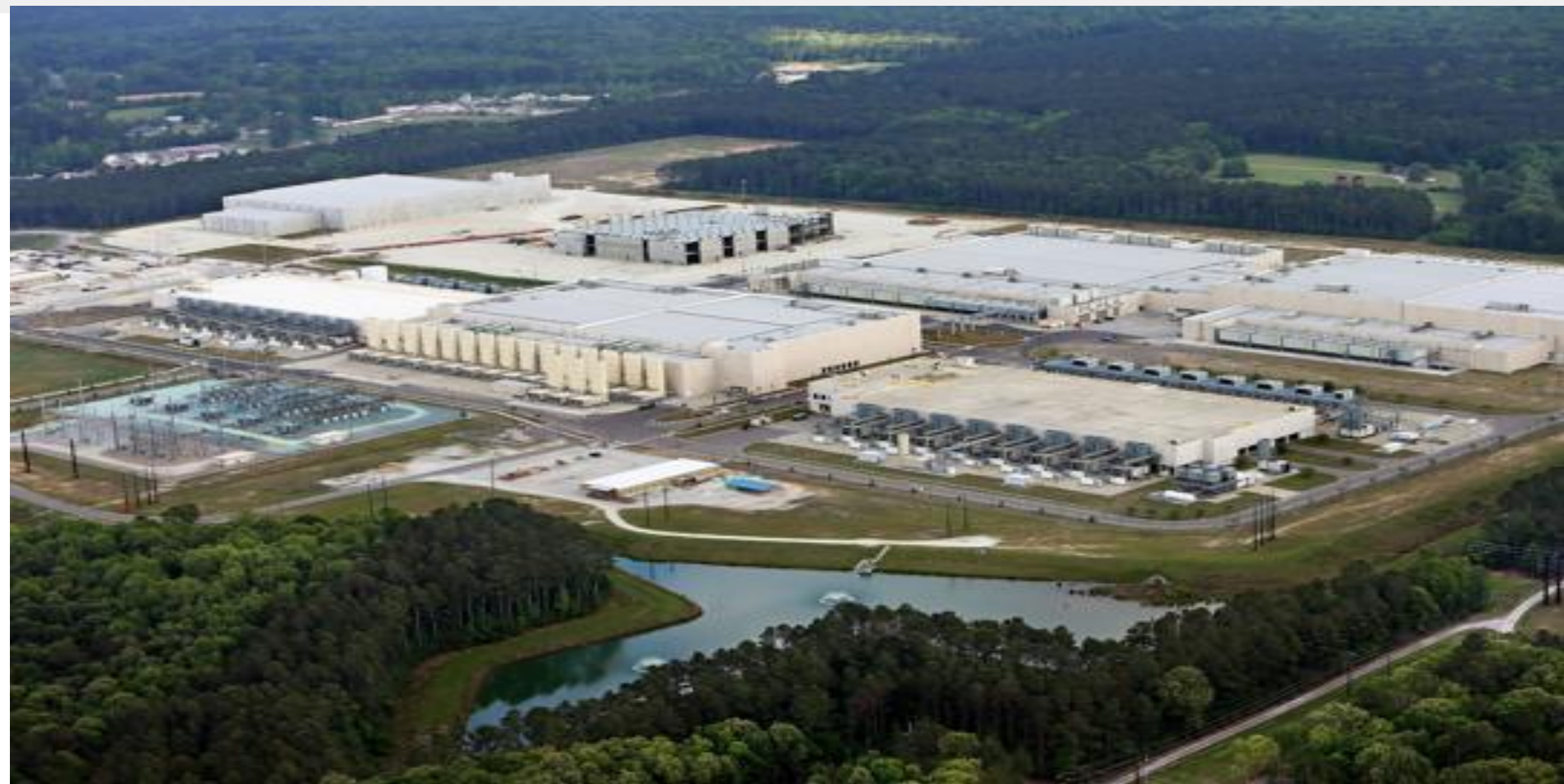
Google Data Center in Berkeley County by Wade Spees wspees@postandcourier.com
